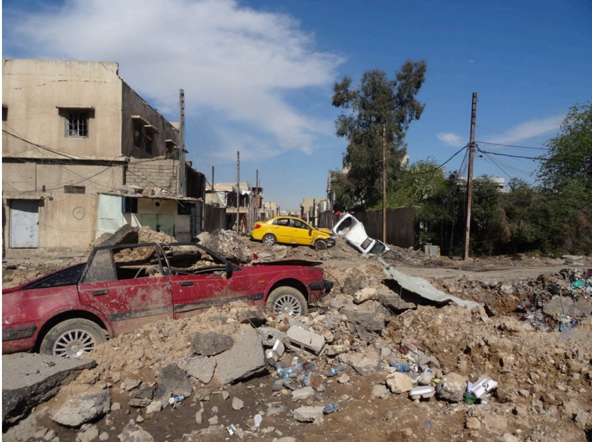
Street in Al Akidat hit by an airstrike and blocked off by vehicles and rubble.
