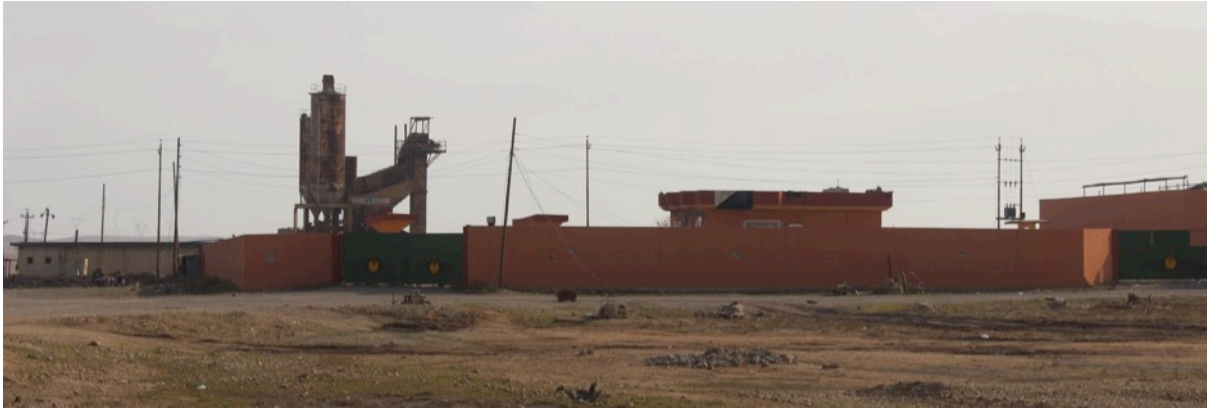
The ISF 9 th Division base from the north.
