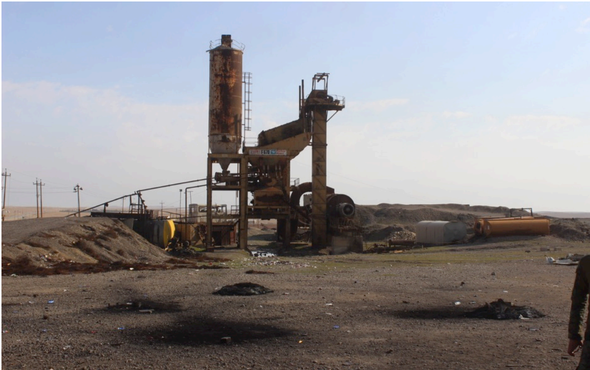
An asphalt plant is located beside the road, next to the reception centre.
