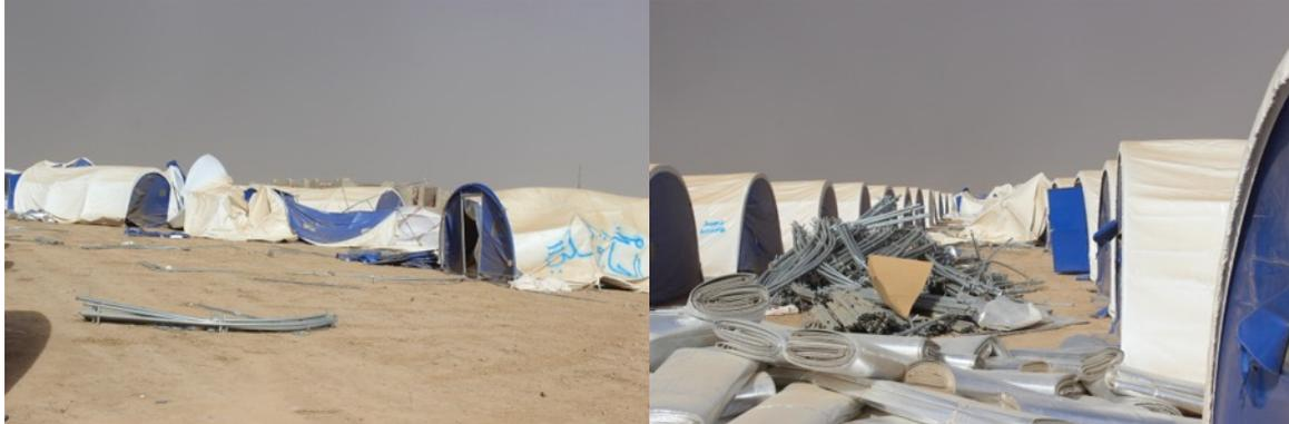
*The 100 unused MOMD tents erected just outside Hasiyah village are in a bad state of repair. It is thought that the damage is due to high winds.*
